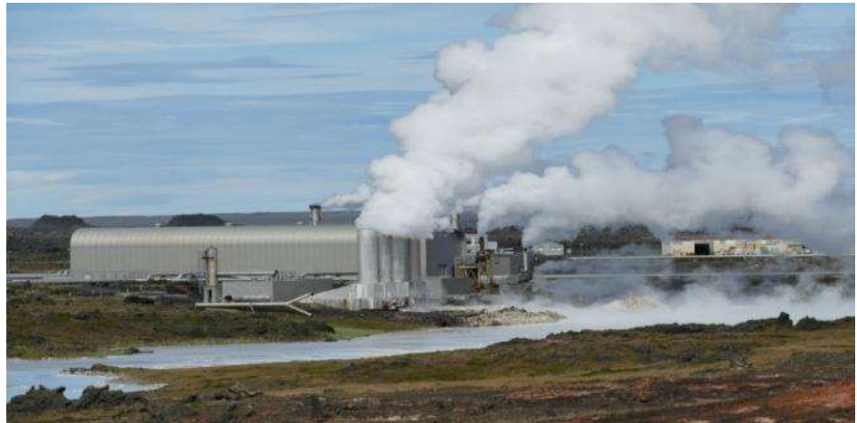
Figure 25. Geothermal power plant.
