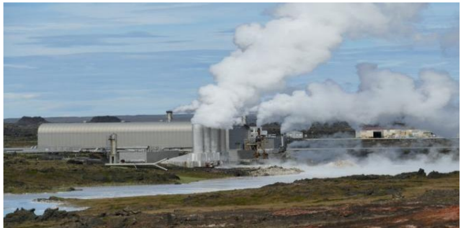
Figure 25. Geothermal power plant.
