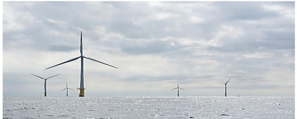
Figure 15. Offshore wind farm.
