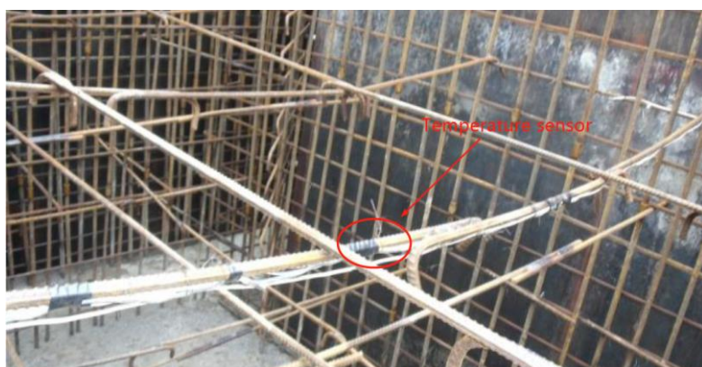
Figure 3. Temperature sensor.
